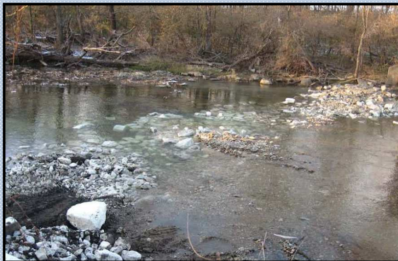
The completed project on the former site of Leonard's Dam in Wilmington, Illinois. As the new stone accumulates biological material, it will begin to look more like a natural riffle.
